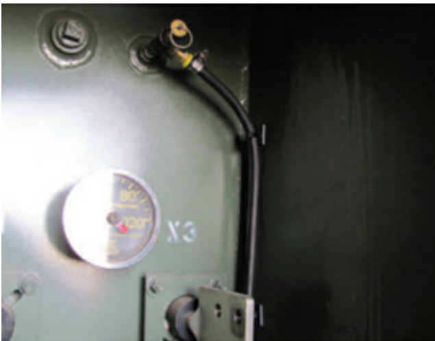
Connection from N 2 Valve to InsuLogix® SSK
