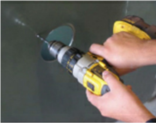
Installer drilling holes indicated on template
